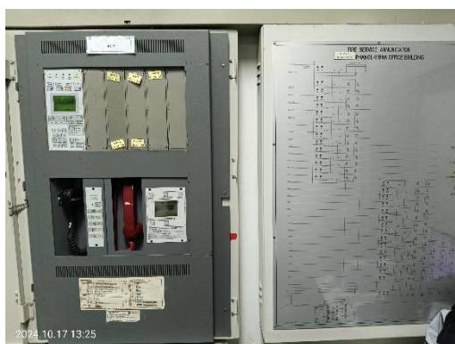
Fire Alarm Control Panel : FCP
